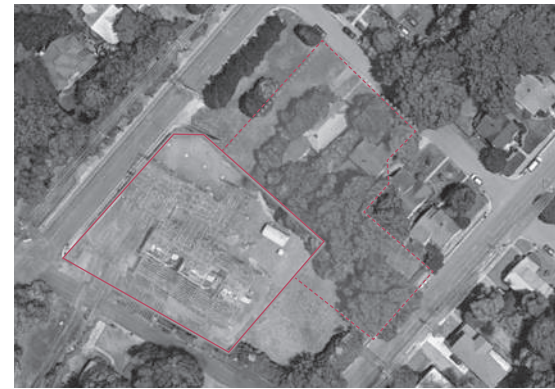
(Above) An aerial view of the Kenilworth substation and the expansion (dotted line) before houses were demolished
