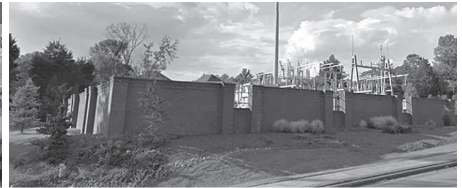
(Above) Brick wall enclosure for a Knoxville substation
