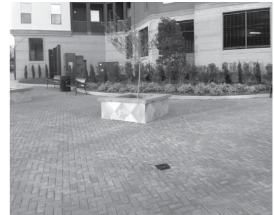
Fig. 1: Empty plaza at Carson Boulevard in SouthEnd. The blank walls and "cars behind bars" strip all possibilities of pedestrian life from this desolate space.
