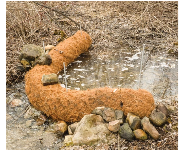
Coir logs are sediment control products made from all-natural, organic coconut. The word "coir" refers to fibers from the outer layer of the coconut fruit.
